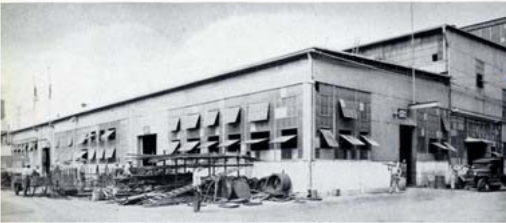
Copper and Sheet Metal Shops
