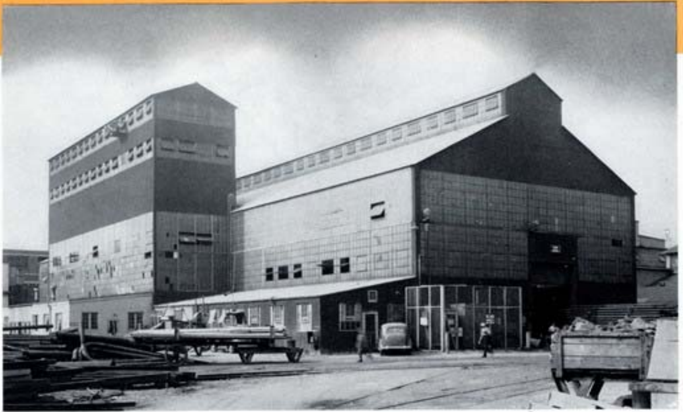
Welding and Fabricating Shops
