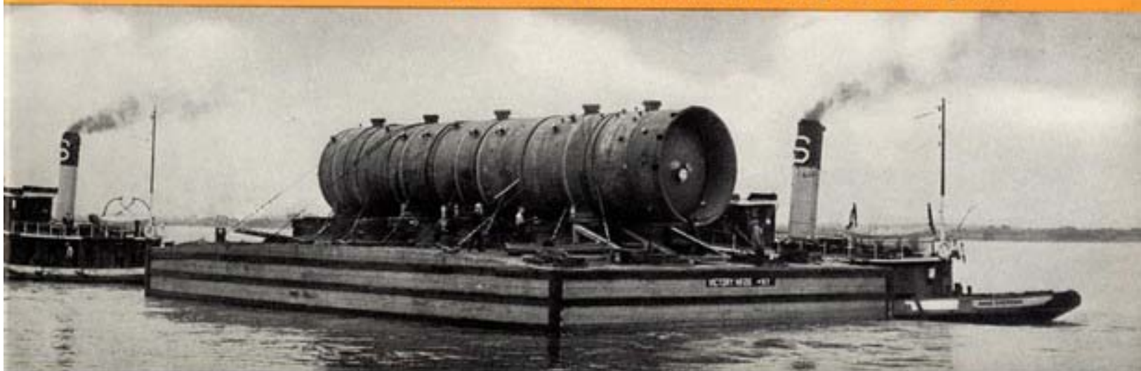
Alloy Lined Reactor, 16 ft. diameter; too large for land shipment.
