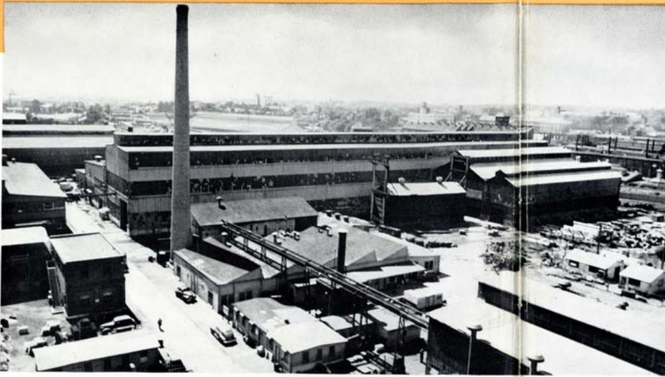
BOILER AND PRESSURE VESSEL SHOPS SHOWING LARGE STRESS RELIEVING FURNACE
