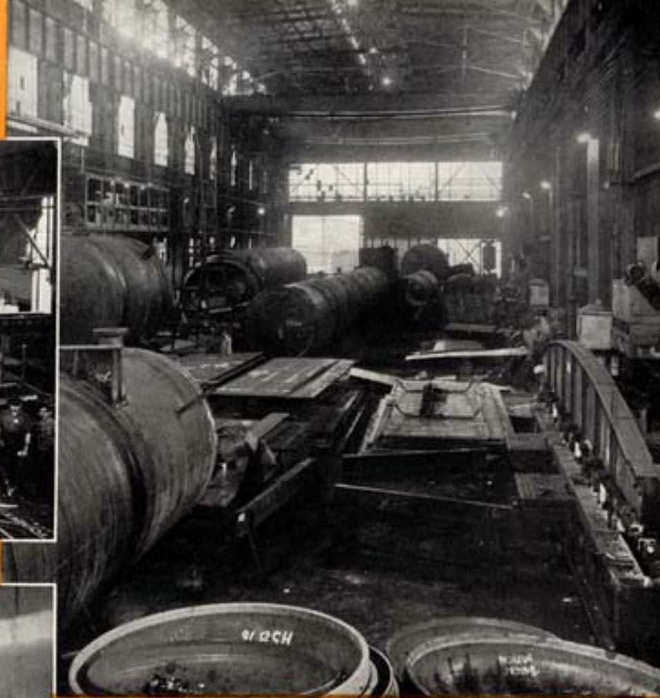
Heavy Welding Section.
