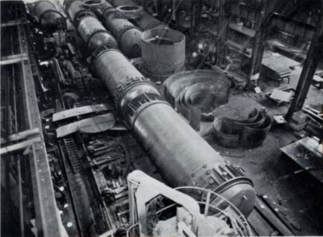
Cracking Cases on Assembly Floor.
