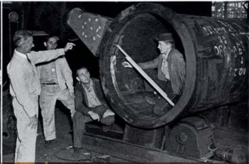
X-raying Special Thick-Welded Sections.
