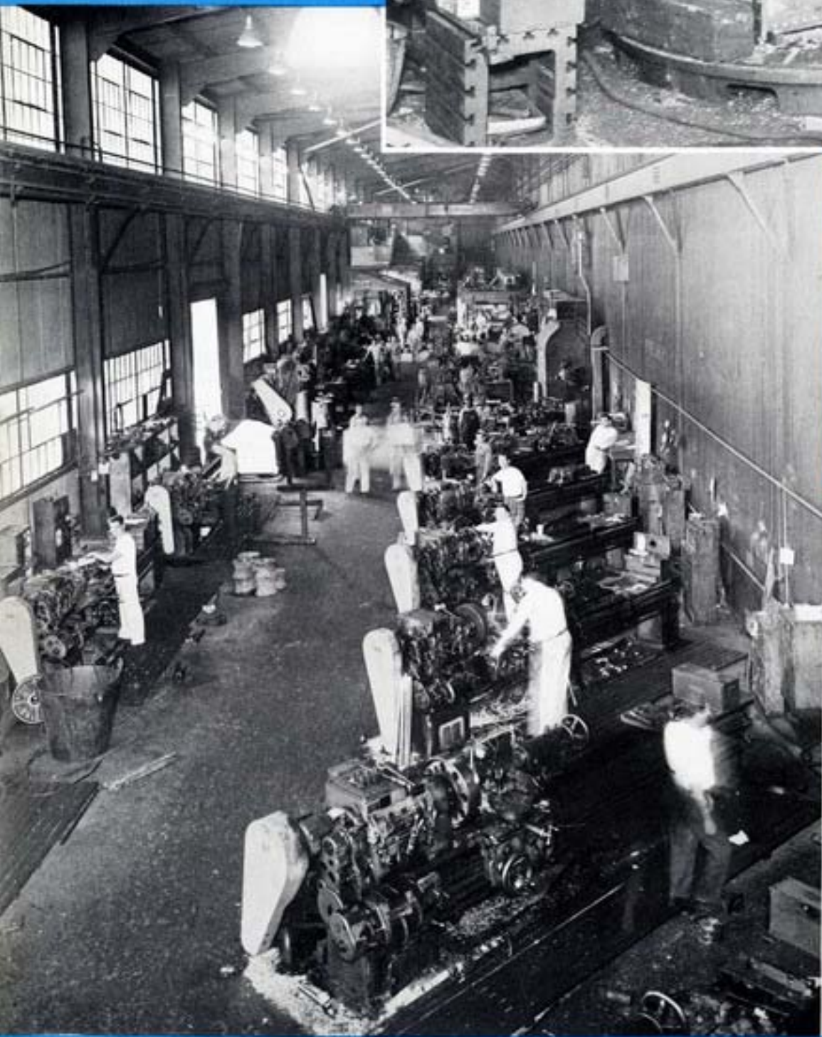
General View of Light Machine Shop.
