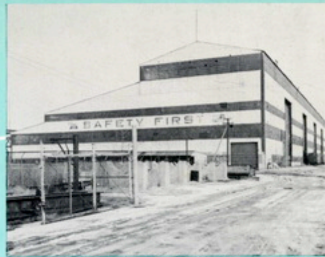
North Yard Fabricating Shop
