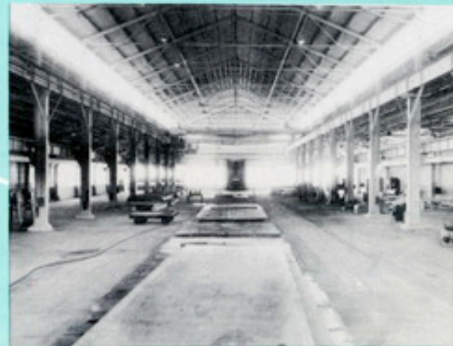
Alloy Steel Fabricating Shop
