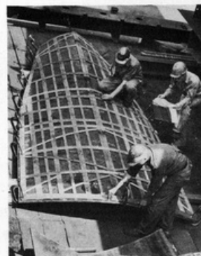
Apprentice Boys Laying Out a Furnaced Shell Plate.
