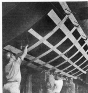
Lifting a Bilge Plate.
