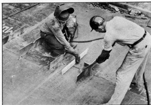
Preparing Deck for Final Welding.
