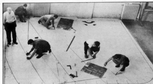
Instructor and Apprentice Boys Working on Body Plan in Shipfitting School.
