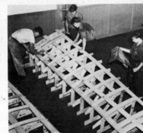
Apprentice Boys Making a Mock-up Mold in Shipfitting School.
