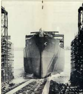
S. S. Elkay — Launched 2:35 P. M. May 30, 1942 — Keel laid January 3, 1942 — Length 300' B. P. — Beam 68' — Depth 37' 9" — Steam Turbine — Built for Seaman Tankers, Inc. — Sponsor: Mrs. Gerald Helmsfeld.
