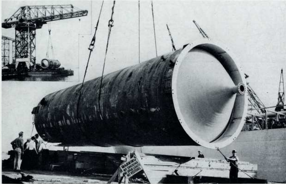
150 TON 16'0" REACTOR BEING LIFTED BY HAMMERHEAD CRANE for shipment from the yard by water, since it was too large for rail shipment. This huge vessel was built in the Boiler Shop and will be used for making aviation gasoline to help win the war.
