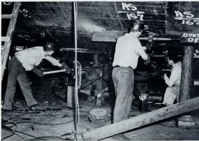
Here we have a 100-ton forward assembly being pulled into proper position by the regulators.
