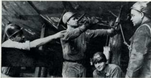
BEN CHMIELEWSKI AND "MOON" BILDER demonstrate the proper way of flushing a bilge seam. Tony DeLilleo, burner, appears well pleased with the burning job. Ed Courtin (left), Assistant Foreman, is directing the job.
