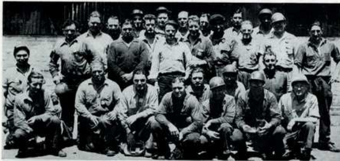
GROUP OF CHIPPERS AND CAULKERS IN THE CENTRAL YARD
