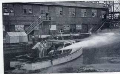
SUN SHIP'S FIRE BOAT, which was bought by the Company through Mr. Carney for the use of the Volunteer Firemen of Sun Ship. The boat is 40 ft. long, has a 7½ foot beam and has a speed of about 12 knots. Installed on the boat are three 500-gallon auxiliary pumps which have a maximum pressure of 250 lbs. Two lines can be run from each pump.
