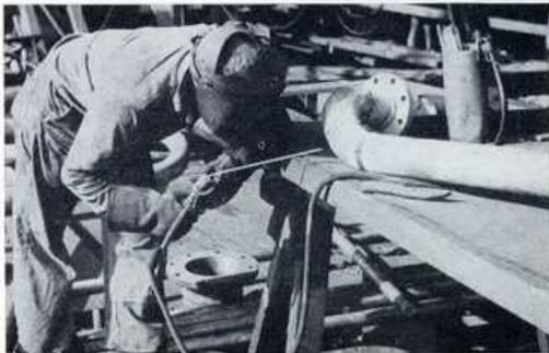
W. HOLLIS welding a butt-weld on pipe.
