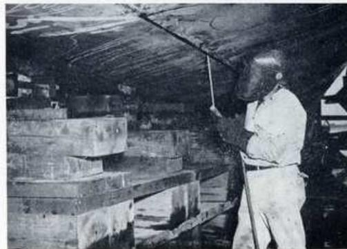
S. FIORETTI backing up a shell seam on bottom shell of a ship.
