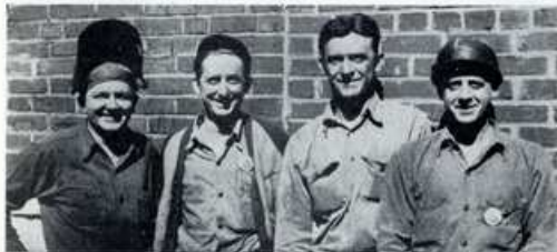
CENTRAL YARD ELECTRICIANS , who make cable racks are, left to right: J. Detesky, 59 dept., Andrew Cassidy, William Helder, and J. Lindenberg, all of 33 dept.
