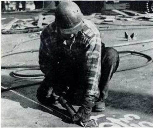
JOE BONKOWSKI preparing a shelter-deck butt for welding.
