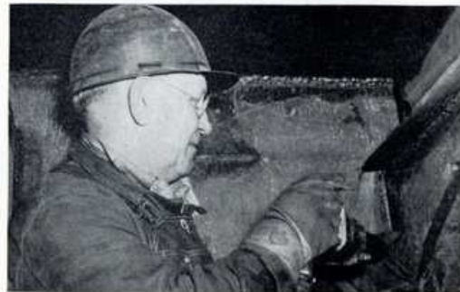
JOHN KREBB stopping a leak on thru-bracket on transverse bulkhead.
