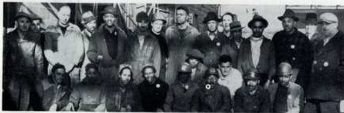
ELECTRICAL MAINTENANCE AND REPAIRS, No. 4 YARD — Left to right, kneeling: J. Patterson, E. Billops, M. Kellum, W. Anderson, M. Selby, C. Campbell, W. Hudnell, J. Fitzgerald, C. Black and T. Smith. Standing: F. Kelly, leader, W. Lallone, R. Hampton, E. Crump, J. Weldon, V. Hutchinson, H. Baldwin, leader, J. Bynum, W. Williams, J. Yocum, J. Page, H. Gregory, J. Smith, J. Heaps, assistant foreman, A. Jenkins, assistant foreman.
