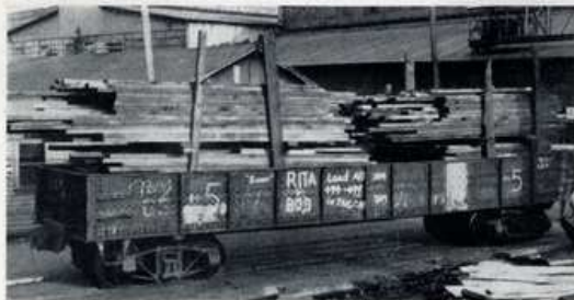
THIS CUMBERSOME, OLD, INEFFICIENT WAY of moving lumber around the Yard has been replaced by the modern ROSS CARRIER which Sun Ship recently purchased as a wartime necessity.
