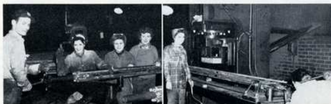
Left to right: J. Triska, removing hydrostatic test connection from tubes on test table. A. Melito, making repairs to weld on the tube. C. Bottino and M. Shaw, Inspectors.
