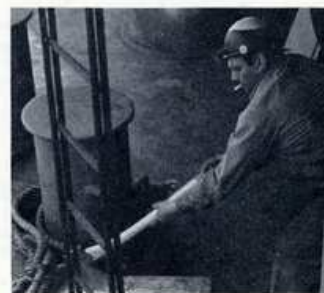
CHARLES FAUST, South Yard rigger, is ready to cut the rope which holds the turning wire on the ship while it is being launched. This wire is attached to heavy anchor cable that lies in the river bottom with the other end of the cable attached to shore. They are used to turn the ship during a launching after it hits the water.
