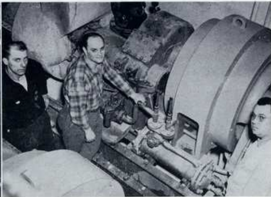
OPERATING THE AUXILIARY GENERATORS which generate electricity for motors and lighting aboard ship. Left to right: Steve Latocha, Assistant Foreman; Joe Meroth, Machinist; Eddie Pack, Machinist.
