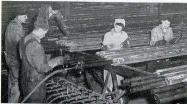
THE TUBE being hydrostatically tested and inspected by Harvey Overline. Helping him are Fred Coldinon, Robert Craig, Judith Judefing and Sophie Hmielefski.
