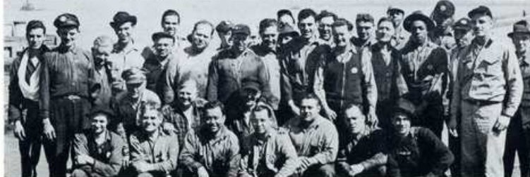
47 DEPARTMENT, SOUTH YARD FABRICATING SHOP, DAY SHIFT
