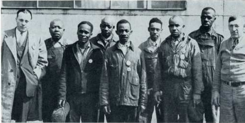
RALPH V. RULON, Inc., PHILADELPHIA, EMPLOYEES who install Mastic Asphalt floor in refrigerator rooms, etc., on all vessels built in Yard. Left to right: P. L. Frazier, Supt.; J. Coleman, R. Waters, W. Gaines, T. Simmons, L. Kellogg, W. Pindell, A. Williams, B. Frank Sheidy, Foreman.
