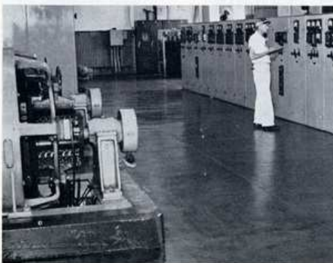
GENERAL VIEW of the Power House.
