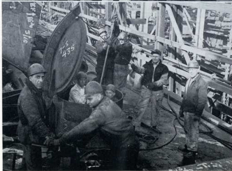
OPERATING ROD BEING LOWERED THROUGH HATCH TO POSITION IN MAIN CARGO LINES by Len Seddon, Jim Hughes, R. Chrystler, E. Brooks, A. Peterson, J. Taylor, Brown, and D. Reese Esrey, Assistant Foreman, all of 36 Department.
