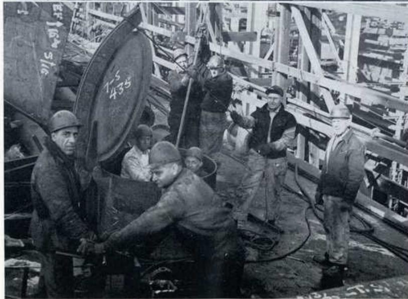
OPERATING ROD BEING LOWERED THROUGH HATCH TO POSITION IN MAIN CARGO LINES by Len Seddon, Jim Hughes, R. Chrystler, E. Brooks, A. Peterson, J. Taylor, Brown, and D. Reese Esrey, Assistant Foreman, all of 36 Department.
