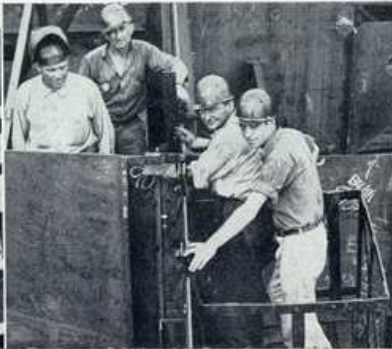
REGULATORS MAKING UP WING bulkhead to longitudinal bulkhead at the after end of midship box. J. Thompson, Ass't Foreman I in charge of shipways No. 17 to No. 20, North Yard; J. Kirinich, Ass't Foreman II; W. Culp, Regulator 1st Class; T. Stephens, Welder.
