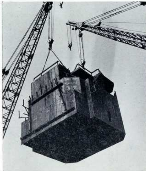
MIDSHIP HOUSE BEING HOISTED to erect on Hull 355. This house was assembled by 47 Department at 29 Bay in No. 4 Yard, No. 4 Yard workers like to boast that it is the largest, most complete midship house erected in one piece in the entire Sun Yards. This lift represents 53 tons and was erected and regulated in about 45 minutes from the time it was hoisted by the cranes. Harry Husum, Erector Foreman, was in charge.
