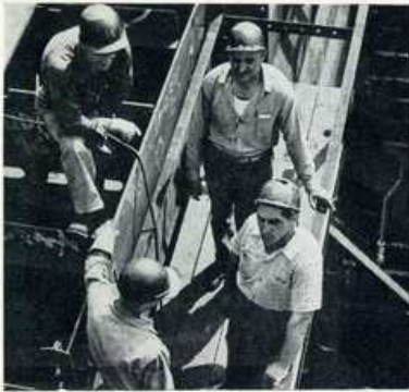
REGULATORS PULLING IN SIDE SHELL to wing bulkhead at the forward end of midship box. T. Marsick, Ass't Foreman in charge of shipways No. 1 to No. 4, Central Yard; T. Saraullo, Ass't Foreman II; E. Blyth, Leader Regulator; J. Kralovich, Regulator 1st class.
