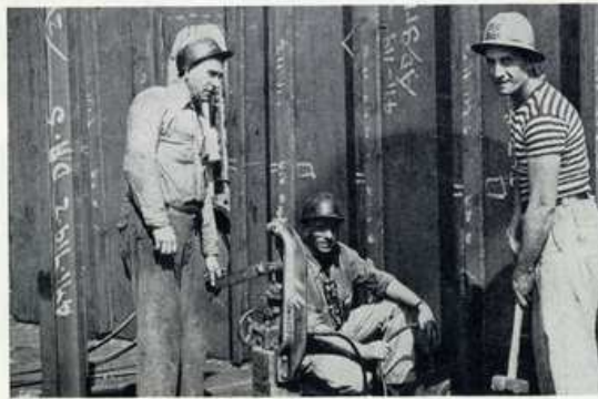
REGULATORS MOVING TRANSVERSE BULKHEAD at after end of midship house to proper set lines of Hull 471. J. Pastick, Foreman Regulator in charge of shipways No. 5 to No. 8, Central Yard; B. Innezelli, Leader Regulator; A. Barbic, Regulator 1st class.
