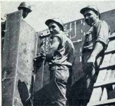
REGULATORS MAKING UP CL BUTT of transverse bulkhead No. 1.20 above 3rd Deck. M. Griceo, Ass't Foreman I in charge of South Yard No. 9 to No. 12 shipways. F. Johnson, Leader Regulator; A. Georgi, Regulator 1st class.
