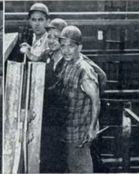
REGULATORS MAKING UP LONGITUDINAL BULKHEAD to C. L. transverse bulkhead on forward end of midship box. Left to right: S. Sherry, W. Stanoski, and J. Santa Maria.
