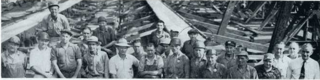
CENTRAL YARD LAUNCHING CREW WHEN THE S.S. MISPILLION HIT THE WAVES
