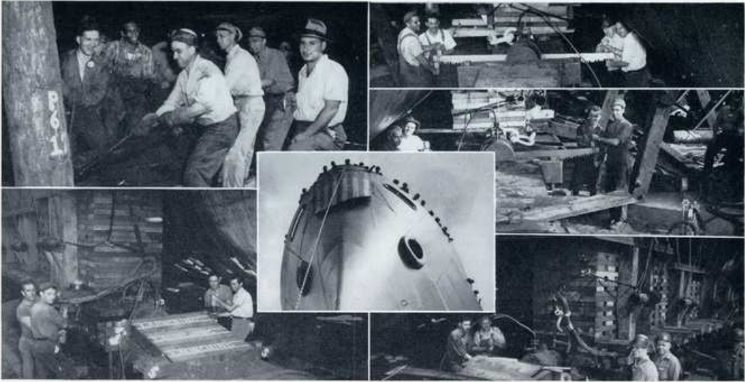
(Upper left) — KNOCKING OUT one of the last supports. (Lower left and right) — THE CUTTING OUTFIT from Central Yard whose saws release the ships.
