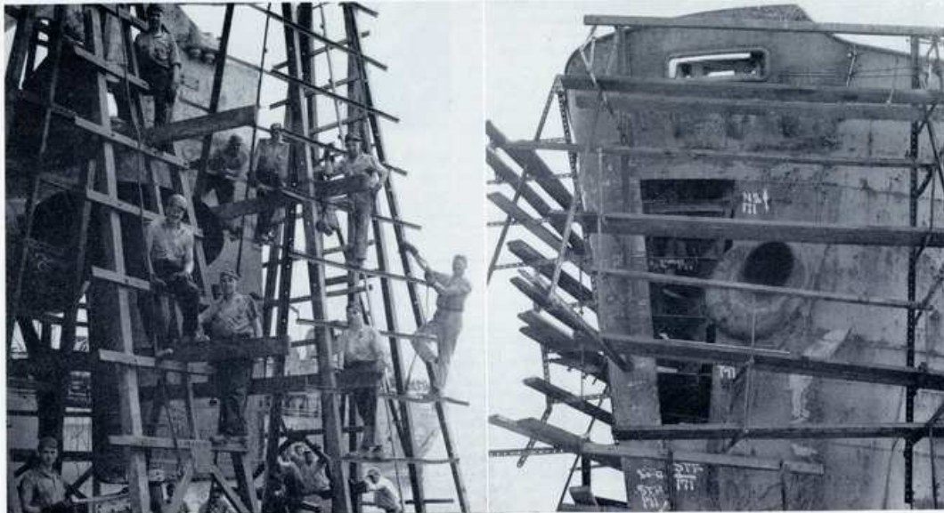
NEW "NOSE" is put on a ship by skilled Sun Ship repair crew. This ship had been in a collision.
