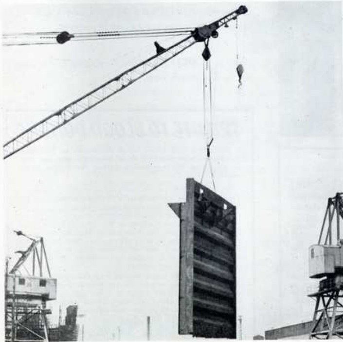
ANOTHER BIG ASSEMBLY is being swung towards the shipway in the North Yard.
