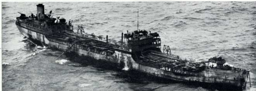
The S.S. MURFREESBORO, operated before the war by Marine Transport Lines, was staunch enough to withstand a convoy collision that resulted in the sinking of the ship which rammed her and to survive the flames that raged throughout her length and on the oil-drenched surrounding sea.
