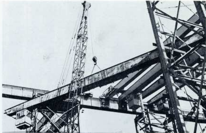
REMOVAL OF A 10 TON CRANE in the Central Yard was a delicate job successfully handled recently. The upper picture shows part of structure being lowered while left the crew that did the work is shown.
