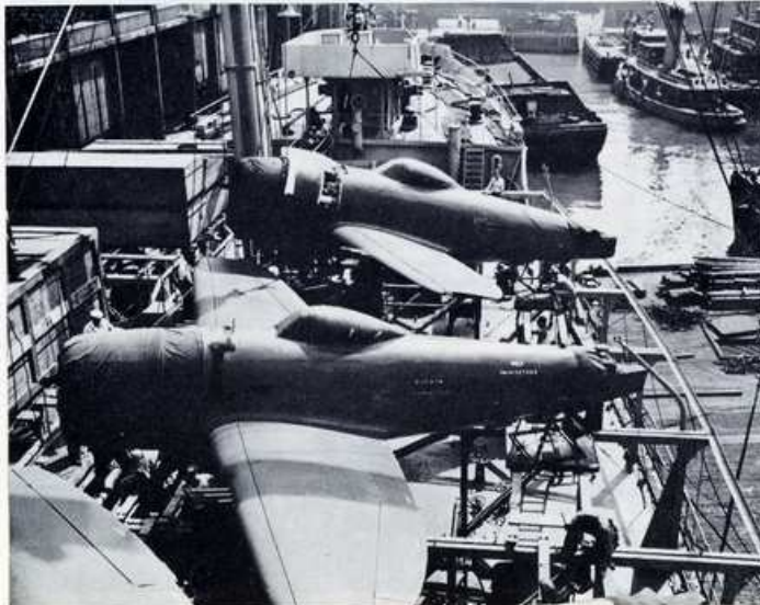
BY USING AN EXTRA EMERGENCY DECK Sun Ship tankers and others were able to carry planes and other munitions in addition to oil and gasoline. They helped speed up the war effort.
