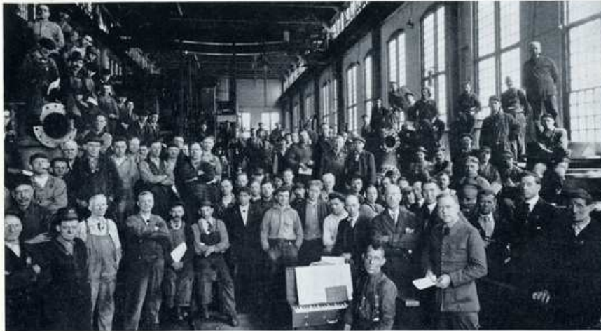
THIS PICTURE OF A BOND DRIVE DURING THE FIRST WORLD WAR was taken in the machine shop at the Wetherill Plant. It was conducted by the representatives from the Y.M.C.A. Some of the Sun Ship employees shown here are still working at Wetherill.
