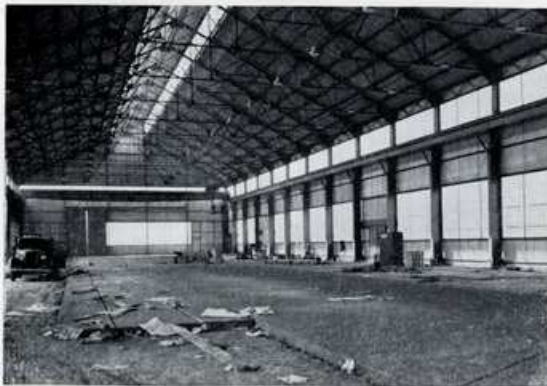
BALL PARK STORAGE BUILDING was constructed in rapid time during the fall of 1941.
