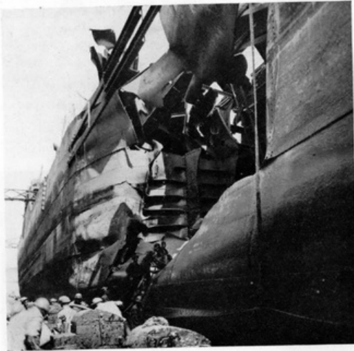
MAJOR DAMAGE to the "Bidwell" was quickly repaired by Sun Ship workmen and the tanker was soon back in service.
