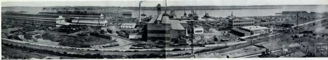
THIS STRIKING PHOTOGRAPH shows the yard as it appeared July 1, 1913. Lines extend from Bridge Creek on left to Parkman-Widener plant, extreme right. At that time there were five shipways. The Dry Dock had not been built although pile driver can be seen on that site. Present South Yard was used for storage. Midway on extreme right can be seen part of the famous "Red Fort", scene of athletic activities. Two wet basins are seen. This photograph was made in the late afternoon and shows workmen leaving the yard at quitting time.
