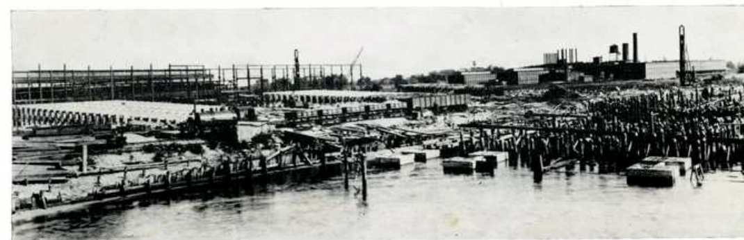
(Below) — SEPTEMBER, 1916 — Notice how the ways are taking form and steel for the cranes is being placed in position.
