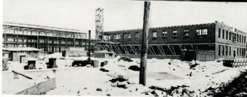
MARCH, 1917 — Cold winter of 1916-17 continues but this month finds the brick-work on the office building completed and steelwork on boiler shop rapidly taking form.
