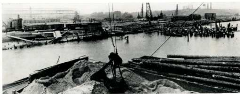
JULY, 1916 — Piles are being driven on the waterfront. Skeleton of Mold Loft is seen in distance. This was Sun Ship's first building.
