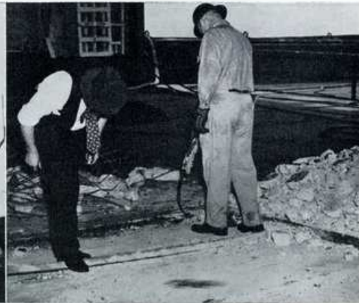
WORKMEN start to remove the concrete from the rails.
