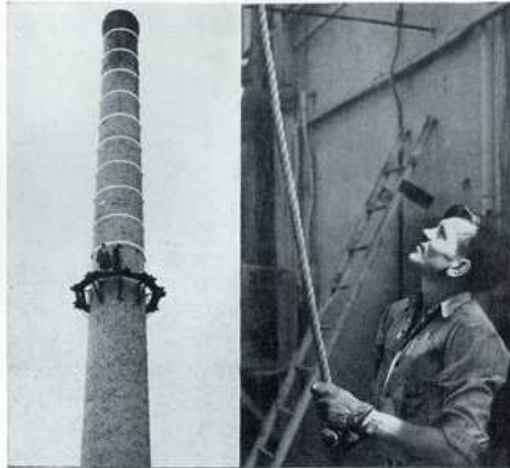
PLACING STEEL BANDS around the upper part of the 155 feet smoke stack at the heating plant was the job for the steeplejacks shown on the scaffolding. They worked from the top down using 11 bands five feet apart. Right, JOHN WELLS of the H. R. Heincke Company, who set the ladders to reach the top of the stack.
