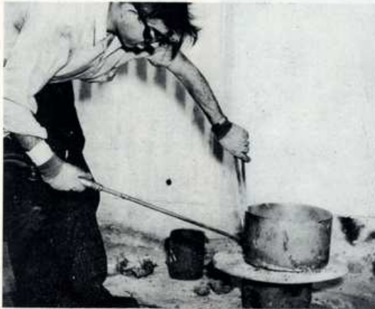
R. SHOEMAKER cleaning a pot with heat and zinc oxide. He was aided by Tom Purcell.
