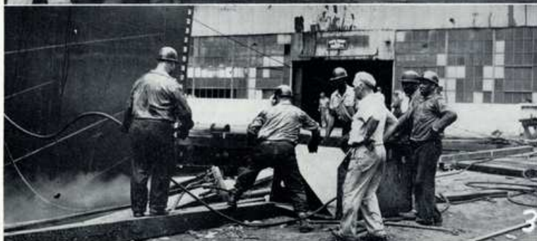
ALBERT BUZA, leaderman in 68 Dept. directs Thomas McGranahan in the cutting of the lashing for the river wire which aids in turning the vessel after she is floated.
