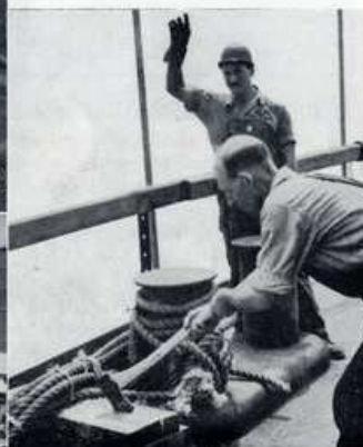
ALBERT BUZA, leaderman in 68 Dept. directs Thomas McGranahan in the cutting of the lashing for the river wire which aids in turning the vessel after she is floated.
