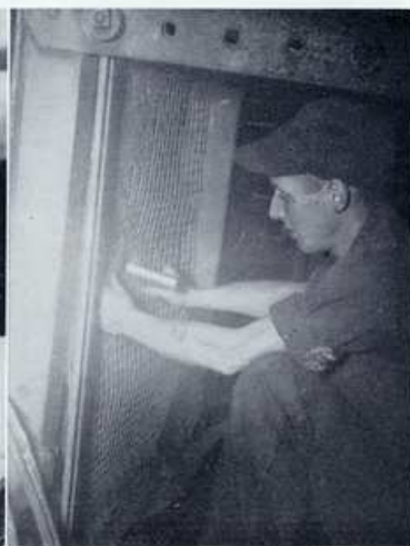
GEORGE BENDITT demonstrates how his hammer is used to straddle insulation pin. This hammer, with a hollow end on one side, has speeded up the work of installing material.
