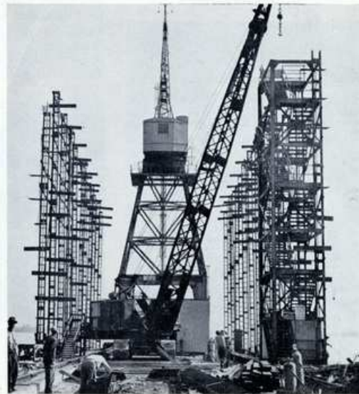
CRANE lifts stair tower from its base.
