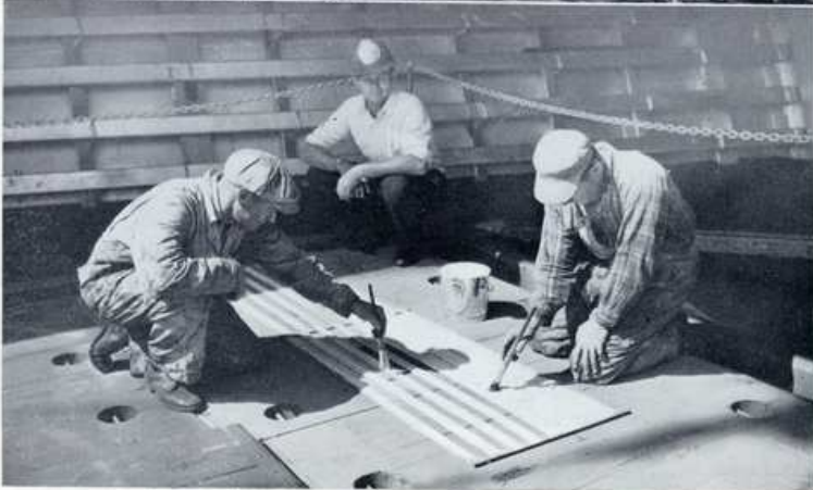
FRED RICHARDSON'S form for putting stripes on hatch covers is simple and speedy.
