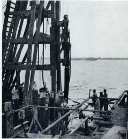
PILE DRIVER is shown sinking a 50 ft. pile into river bottom.
