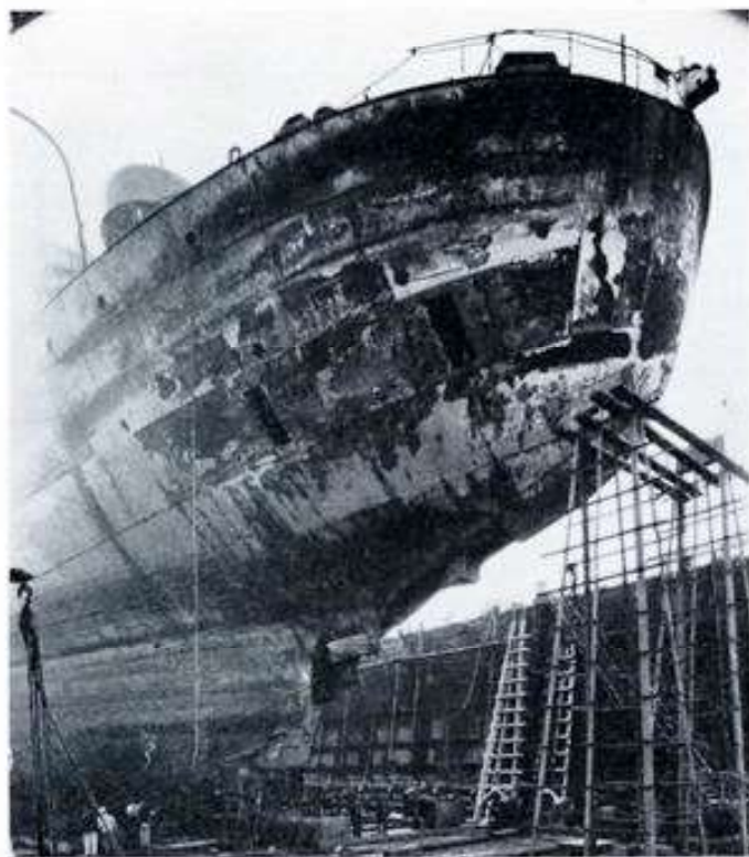
THE "FLORIDA" when she came to Sun Ship for repairs with rudder and propeller gone after being torpedoed.
