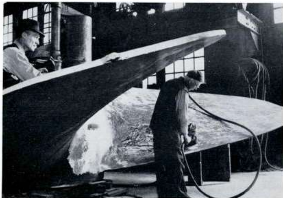
MEN AND METAL is the title of this photographic study at the Wetherill Plant. Otto Leinhauser, foreman, and William Bilsky, grinder, are working on a manganese bronze propeller wheel that shimmers like gold in the shop shadows.
