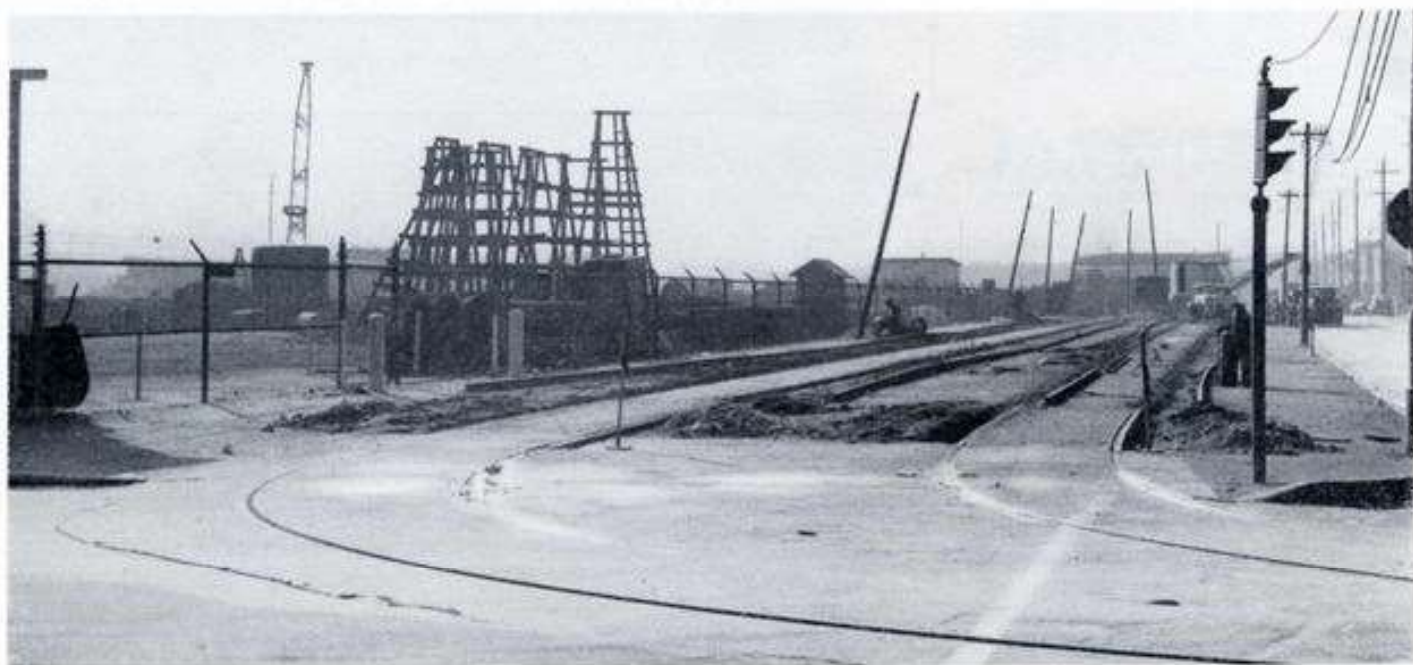
This picture shows removal of the trolley tracks.
