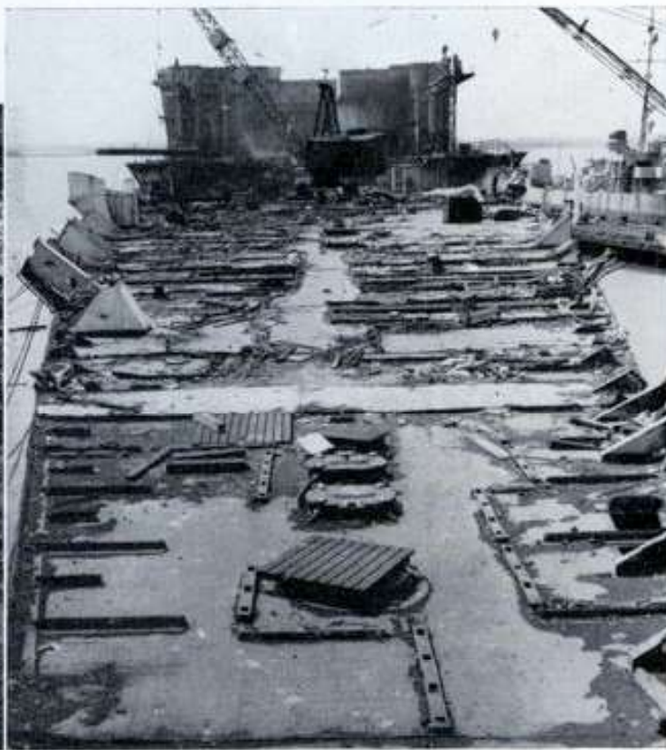
AIRCRAFT CARRIER CASABLANCA arrives at North Yard and joins the RANGER and other scrap ships. Lower view shows deck of RANGER (right) and GOVERNOR COBB (below) with work of demolition going on rapidly.
