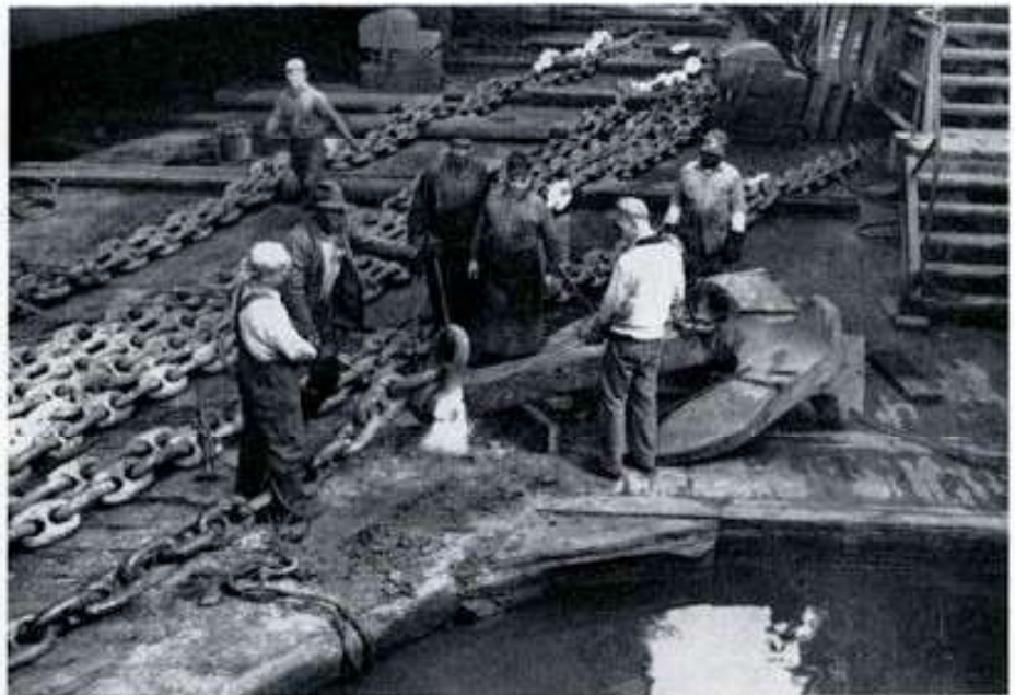
EVERY NOW AND THEN the shackle on a ship's anchor becomes loose and must be hardened up. Here is an outfit on the job. After the metal is heated, sturdy men with sledge hammers do the rest. Note the hundreds of feet of anchor chain on the floor of the dry dock.
