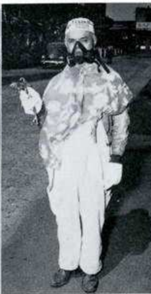
A CHEMICAL CARTRIDGE RESPIRATOR with G. M. A. cartridge is used when the liquid vehicle or the solvent used in the paint is injurious to the health.
