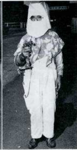
A PAPER HOOD , supplied with compressed air of sufficient pressure to prevent outside spray from entering it, is used under all conditions where it is not too cumbersome.
