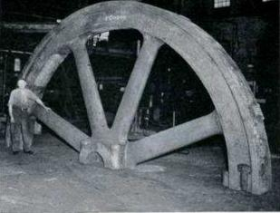
THESE TWO PICTURES WERE TAKEN AT THE WETHERILL PLANT and represent important castings in a large Carliss engine. The casting weighs about 38,000 lbs. On the right is a casting of one half of a
