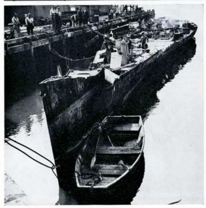
AFTER ALL DECKS had been removed and all partitions knocked out, the frigate BEAUFORT was then sent to No. 7 Way, Central Yard far the final work of demalition.
