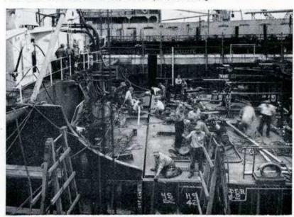
LAST ACT IN RECONSTRUCTING THE AVILA to carry propone gas was welding the brand new midsection and the stern section together for the final welding operation. Photograph shows how accurately Sun Ship engineers and mechanics had planned and executed the big job of cutting a ship apart to lengthen and modernize it.
