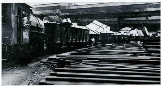
HERE ARE FIVE CARS filled with scrap steel in assorted sizes. Huge assemblies will be cut down to smaller sizes and then shipped to blast furnaces. Trains of 5 and 6 cars are now common in the Yard.
