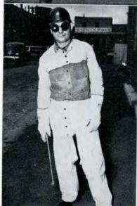
MICHAEL OLANIN, 60-38, SUN SHIP BURNER for the past 18 years demonstrates the proper protective clothing that should be used when burning in the open and in confined spaces, hard to ventilate:
