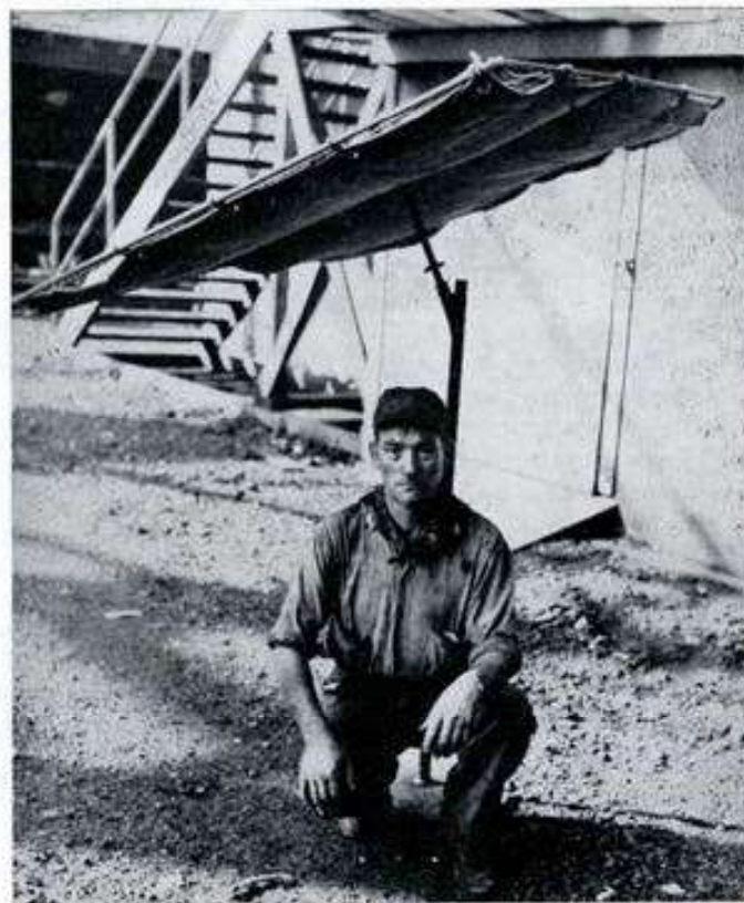
DURING the past two summers, Welders and others working in the sun have used these shades designed by the Safety Department.
