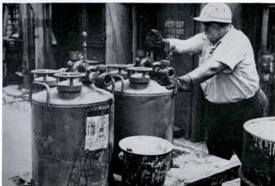
FIRE MARSHAL JOHN OGDEN is testing out Foamite fire equipment to be installed on Dry Docks and other places.
