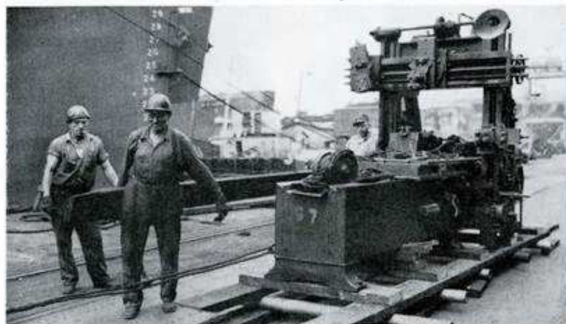
LARGE PLANER, shown in this picture, was hauled from the old 36 Machine Shop completely around the building to be installed in the new addition formerly occupied by the Electrical Department. Workmen are shown carrying heavy planking over which the rollers travel.
