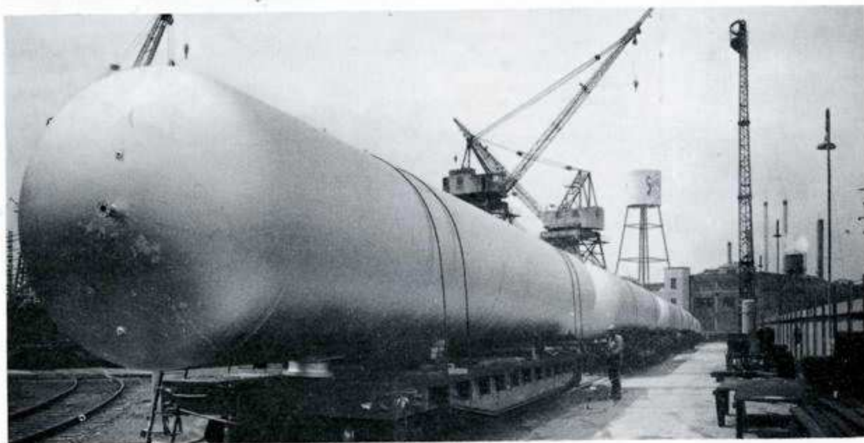
(Below) — HUGE PROPANE TANKS pouring out of our plant. 30,000 gal. capacity of each tank. A single tank holds 24 hr. supply of gas for a city of 70,000 (size of Chester, Pa.)
