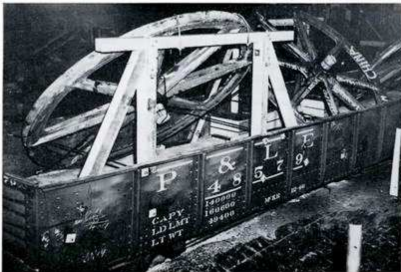
THREE BIG PULLEY WHEELS have been sent to China from our Wetherill Plant. They are to be used in modernizing a mine and will be driven by a 1200 H.P. motor. Each wheel has a diameter of 12 ft. 9 in. and weighs approximately 8000 lbs. They were built on order of U.N.R.A.
