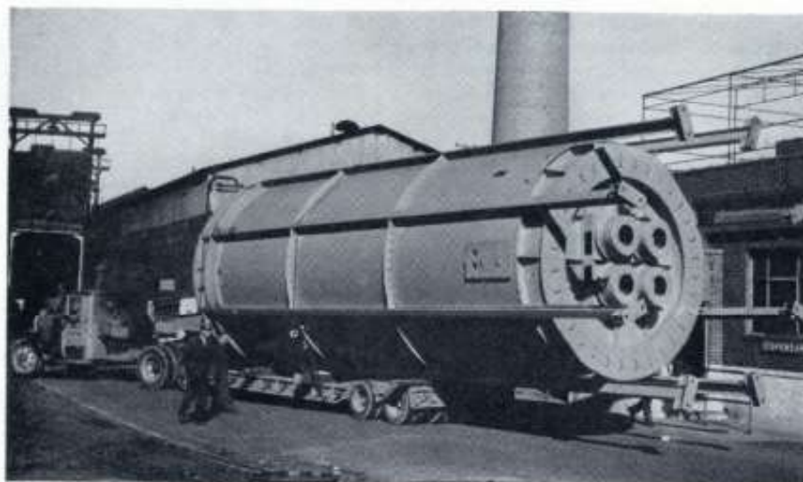
LARGE OIL REFINING VESSEL , 13 ft. 2 in. o.d. 66 ft. high, being trucked from the Yard in section. It was built in 47 Dept. There were several on order and one yet to be shipped.
