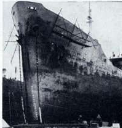
M.S. "STAR BETELGEUSE" ex "Mormaclark" — Built as Sun Hull #180. Purchased from the U.S.M.C. by Compania de la Paloma for operation by Swedish interests. Was towed to the shipyard from the laid-up fleet in the James River for complete examination and overhaul of machinery, removal of Navy installations, drydocking, painting and miscellaneous repairs.
