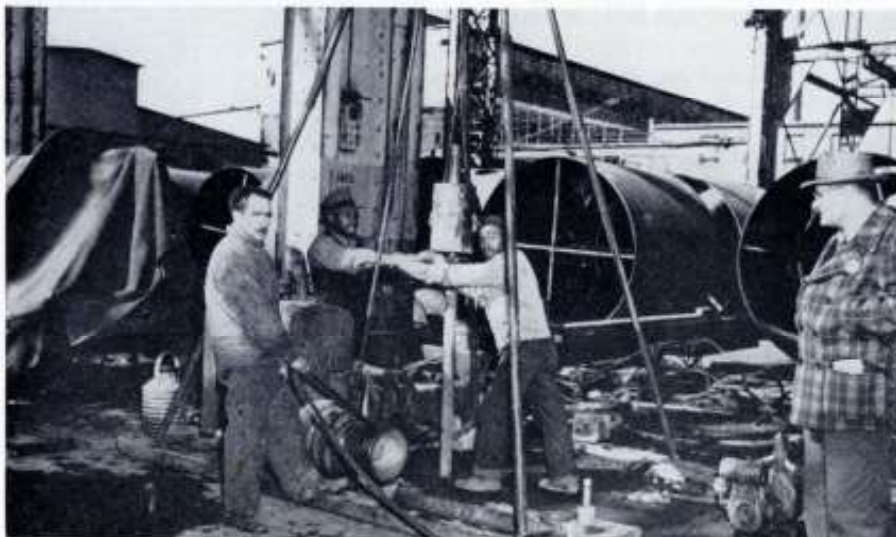
TEST BORINGS being made at No. 1 and No. 2 shipways attracted much interest recently. They were made to determine the depth at which solid rock is to be found along the waterfront in case of any future extension of the shipways.
