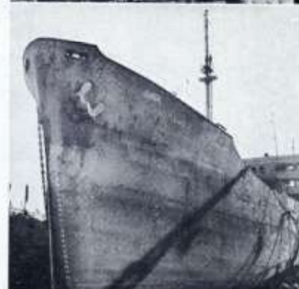
S.S. "VICTORY LOAN" — T2 Tanker purchased from the U.S.M.C. by the Overseas Tankship Corporation. Removal of defense features, drydocking and installation of shell straps.
