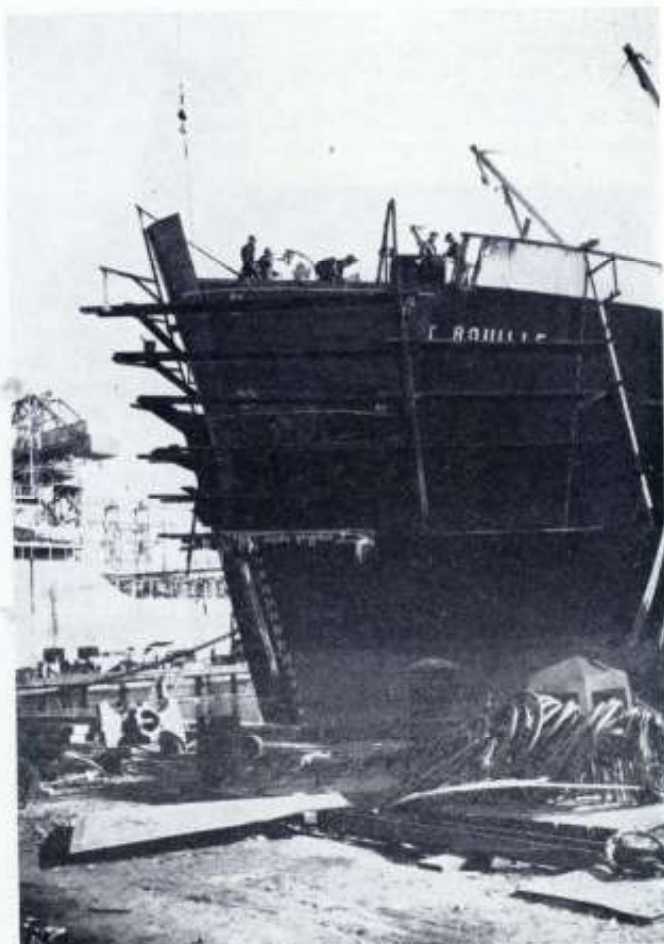
S.S. "FORT ROUILLE" — British cargo ship. Came to shipyard for bow damage repairs on miscellaneous heavy weather damage repairs.
