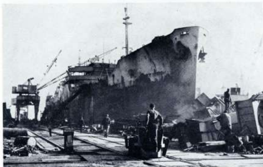
S.S. "WARRIOR POINT" — T2 Tanker purchased from the U.S.M.C. by the Overseas Tankship Corporation. Removal of defense features, alterations to quarters, drydocking and installation of shell and deck straps.
