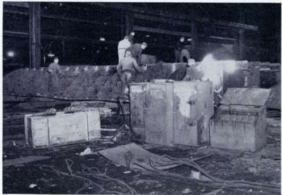
WELDERS and others busy on one of the assemblies for the dredge.
