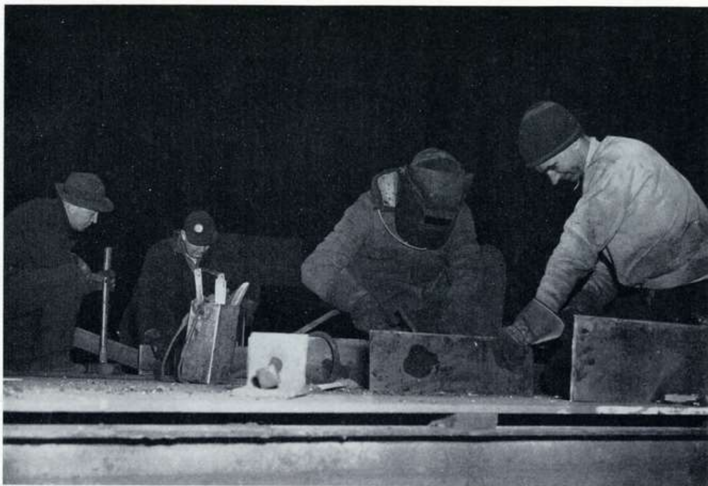
INTENT upon their work these Sun Ship workmen didn't know they were being photographed. They are employed on an inner bottom for a dredge assembly.
