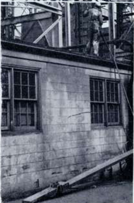
PAINTING SHIPWAYS is a lofty as well as colorful task. Here you see two painters at the top of No. 1 structure. Paint is hauled up to them by men on the ground or lower buildings. It will take many weeks to complete the task of repainting all the shipways.
