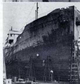
(A) — M.S. "TAMPA" — Norwegian flag cargo vessel on No. 2 Drydock. Vessel came to the shipyard for drydocking, painting and miscellaneous voyage repairs. Clevers are shown at work on the staging for painting. (B) — S.S. "LOUISIANA" — T-2 tanker owned by The Texas Company — Built by Sun Ship as Hull No. 333 (Kernstown). Vessel was completely overhauled, extensively scaled and painted. (C) — S.S. "HELLENIC SKY" — Liberty type cargo vessel owned by the Hellenic Lines, Ltd. This vessel was drydocked, hull cleaned and painted, damage repairs carried out and the vessel returned to service. (D) — S.S. "GULF MARACAIBO" — Tanker built by Sun Ship as Hull No. 233 and owned by the Gulf Oil Corporation. Vessel was drydocked, cleaned, painted and repaired. (E) — S.S. "SENECA CASTLE" — T-2 tanker owned by the Overseas Tankship Corporation. Installation of six rivetted straps on the shell, complete overhaul of machinery and boilers, hull repairs. (F) — M.S. "TIDAROLM" — Swedish cargo ship owned by the Swedish American Lines. Drydocking, cleaning, painting and miscellaneous hull repairs. (G) — M.S. "LIDVARD" — Norwegian cargo ship operated by the Wm. Wilhelmsen Lines. On her second visit to the shipyard within a year the vessel was drydocked, painted, shell and tank repairs carried out. (H) — S.S. "CHARLES SUMNER" — Liberty ship owned by the Seward Line, Inc. Vessel was drydocked, completely painted from the keel to the rail, tailshaft drawn for examination, rudder reinforced. (I) — M.S. "BIDWELL" — Tanker owned by the Sun Oil Company. Radar installed. On this tanker the tailshaft was drawn for examination, one new propeller blade installed and miscellaneous engine, piping and hull repairs performed. (J) — S.S. "ATLANTIC REFINER" — T-2 tanker owned by The Atlantic Refining Company. Built by Sun Ship as Hull No. 488. Annual machinery and hull work performed. (K) — S.S. "ALABAMA" — T-2 tanker owned by The Texas Company and built by Sun Ship as Hull No. 453 (Hubbardston). Complete overhaul of machinery, piping and equipment. (L) — S.S. "SANTA FE MILLS" — T-2 tanker owned by the U.S. Maritime Commission, drydocked for examination. (M) — M.S. "AMERICA SUN" — Tanker owned by Sun Oil Company built by Sun Ship as Hull No. 196. Radar installed.
