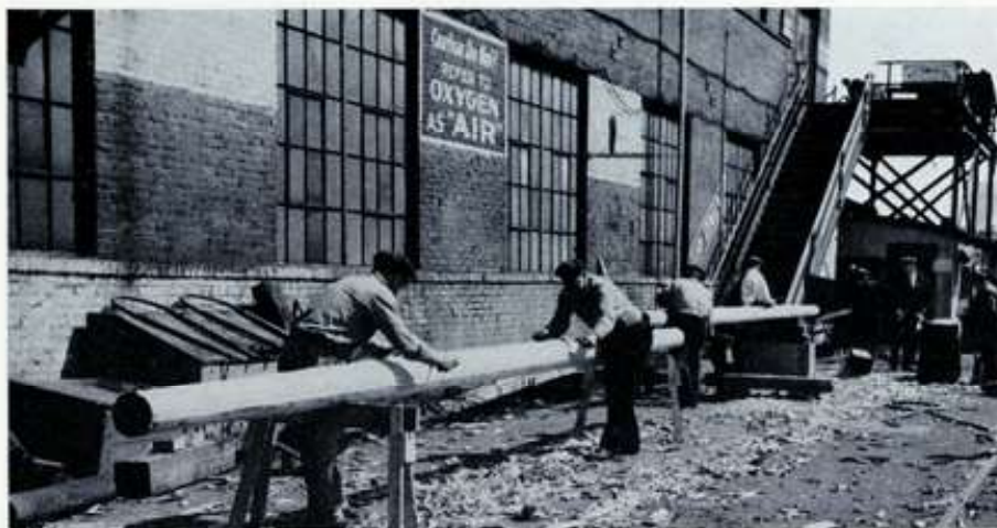
DAYS OF WOODEN SHIPS were recalled recently when the Carpenter Shop made two wooden cargo booms. Mechanics are seen shaving the fir logs to size.
