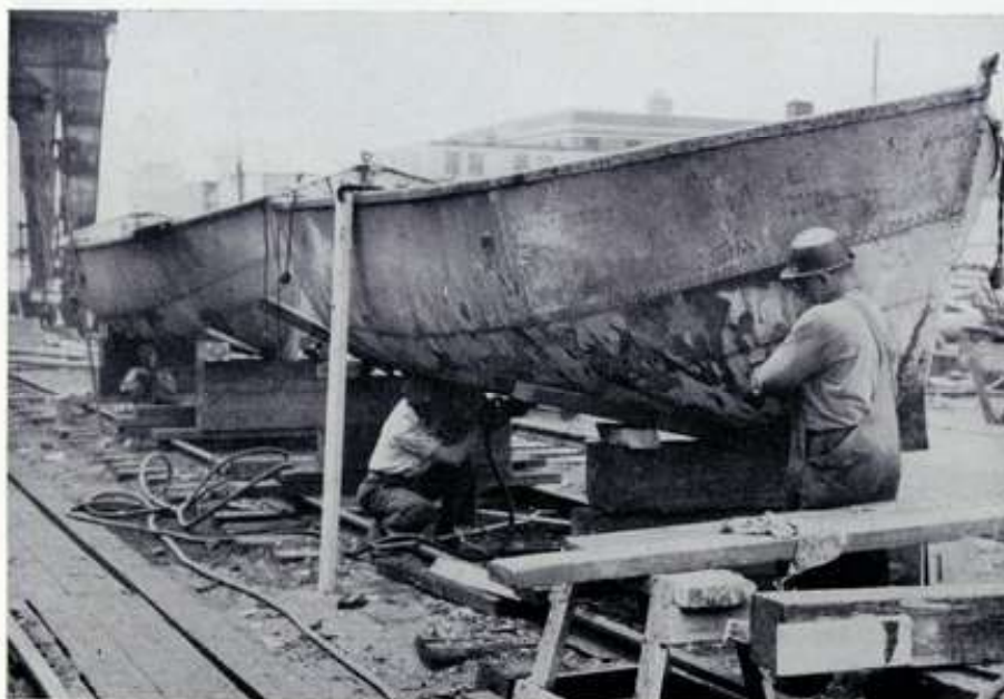
SHIPS' BOATS ARE REPAIRED by Yard workmen who remove dents, fix breaks and restore the small craft. Picture shows two lifeboats being reconditioned.
