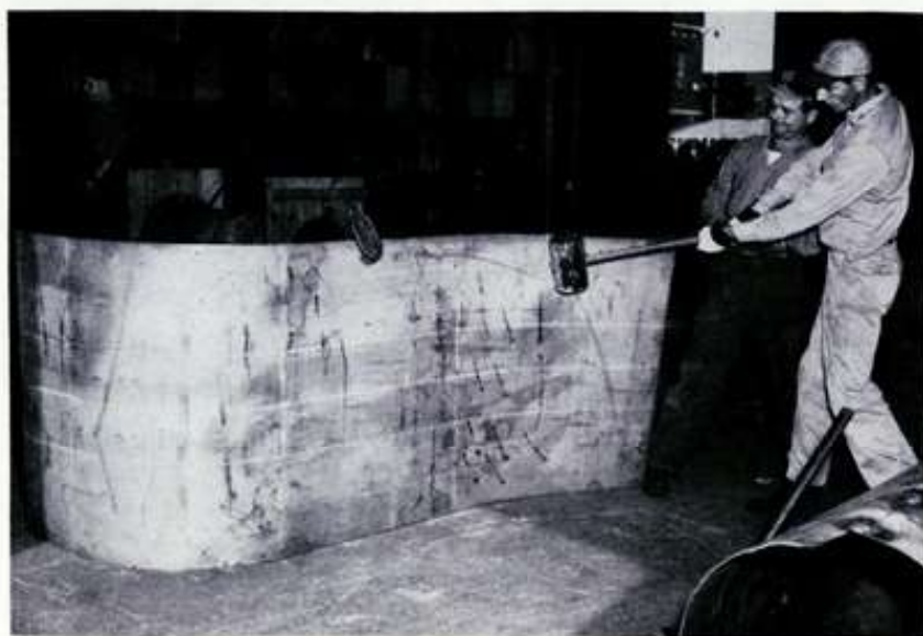
COPPER PIPE with a diameter of more than two feet is one of many big ones for the super-tankers. This pipe is for the main circulating pump. In upper picture Foreman Adam is shown with C. Bauer, coppersmith, and J. Simmons, apprentice. Lower: A. Adam, Jr. and H. Mundle shaping a pipe from sheet of copper.
