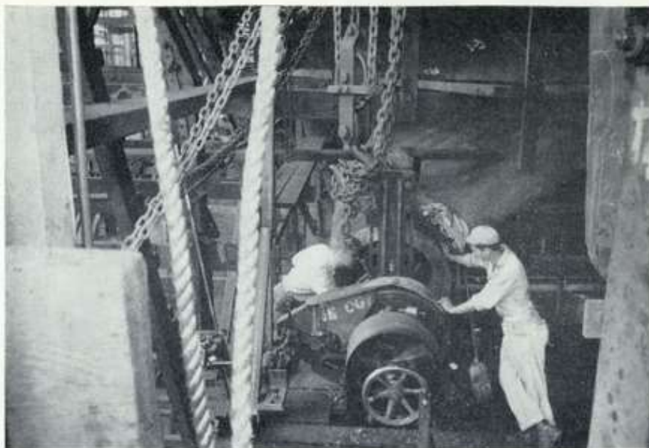
(Above) HORIZONTAL BORING BAR boring fit in spectacle frame for the port stern tube.
