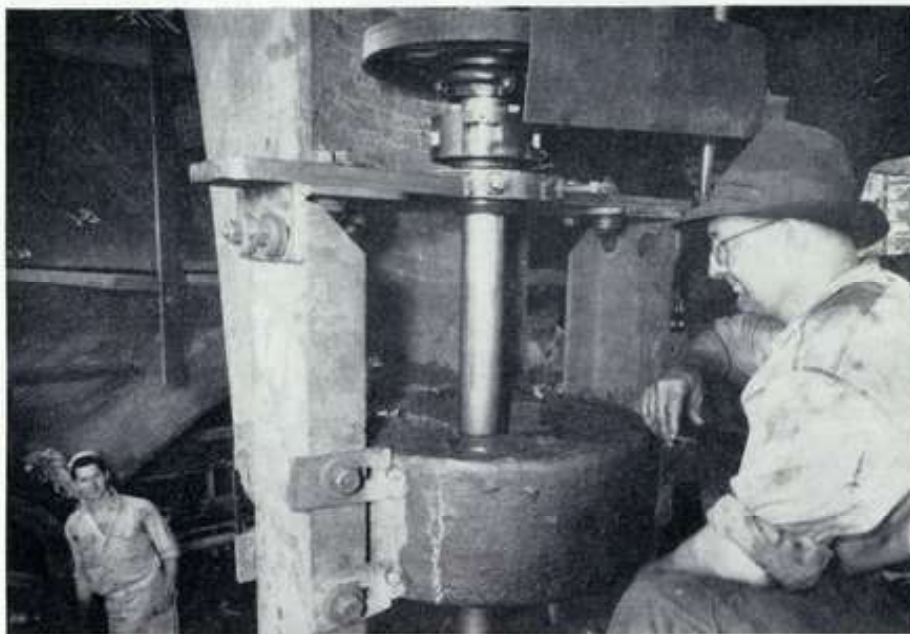
(Lower) VERTICAL BORING BAR boring the gudgeon in the stern frame for the pintle which carries the rudder.
