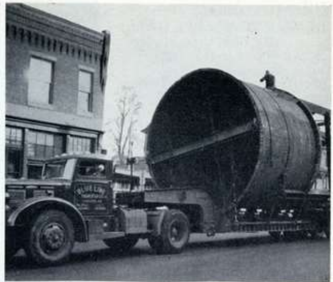
THIS LARGE VESSEL with a 15 ft. diameter was built in 47 Department. This vessel is used by Sun Oil Company for wax refining process. Although this tank weighed about 25 tons, it was hauled by truck from our shop to the job site by a Blue Line truck.
