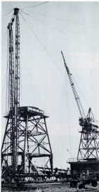
TOWERED MAST AND BOOM used in dismantling Shanty cranes in New York. It paid for shipment to New England. Consider time from top of mast held the shanty but strong standards nearby. One of the Shanty cranes will be driven in distance, another is partly dismantled.
