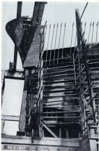
NEW ASSEMBLY being swung into place on a ship under construction always is an interesting sight. The photographer caught this picture recently on this ship.
