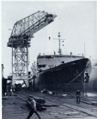
HOISTING OF THE NEW SHIPMAKER'S SHIP is done in conjunction with ship in the basin. From the ground to the bottom tip of the crane is approximately 120 feet. There is a clear area of 30 feet under the beam.
