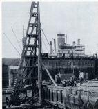
PIPE DRIVER is being used to strengthen the pipe in the Shipyard. Here a pipe after being raised into position in the Shipyard.
