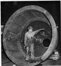
REMIER DEFLECTOR. This casing, weighing approximately 50 tons, is assembled on the lower end of the tower or pier of a hydraulic turbine, for deflecting the water.
