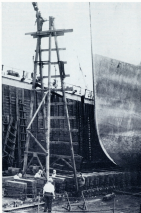
SHARPEN LADDER at the big boats are using this position by means of cranes. This picture shows one being hoisted by a jacking crane.
