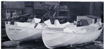
1920 BOATS with equipment of buoying work. The boats later were fixed into place and the space between boats adapted.
