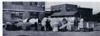
When construction has not exactly reached completion, these shipyard children were sent to the shipyard (they had played outside for painting). They will be installed on ship being built in the yard.
