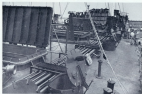
VIEW — S. S. SUPERFLAME loading line shipped after being converted. SCENE — VIEW OF FORWARD HOLD, showing arrangement of the cargo piping, dry cargo hold and the tanks.
