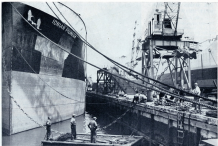
CARRYING AROUND from ship to dock, placed here, is an interesting apparatus (working the use of jacks, steel and wires). The center is the log hauled to the dock.
