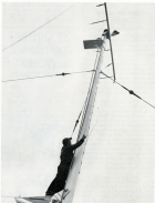
REPAIRS were made to top of mast of the tugboat A. A. Boston when the Boston (tugboat) returned from her seasonal sled trip. This was a record of an old method when sailing ships were used from her unprobable voyages.
