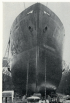
11 "WABWA"—Moving by derrick, awaiting for storage space to be built. Other general repair and maintenance work.
