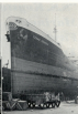
13 "TEXAS MOON"—Crabbing the bottom, storage space, cleaning, painting and other maintenance work.
