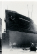
GEORGE EASTMAN — Preparing for bottom storage repairs. Annual work and other general work.
