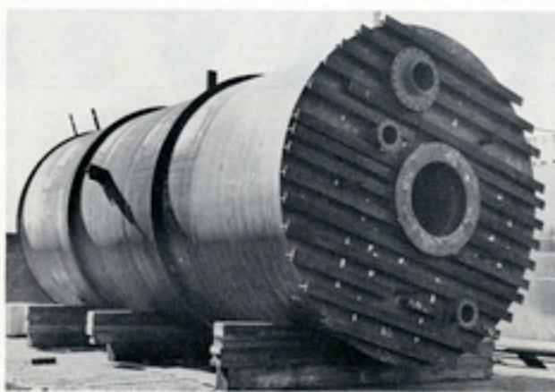
SPECIAL SURGE SEPARATOR VESSEL which was built for the Socony Vacuum Oil Co. at Paulsboro, New Jersey. This vessel is filled with complicated internals. It was too large to ship by rail, therefore, it was shipped by barge across the river. The vessel was built in the Boiler Shop.
