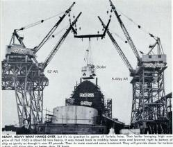
6.2 Photo showing 'Lower Bow' assembly being moved into position on our Hull 610 by four R-25 gantry cranes (ship to be named the SS 'Pennsylvania Sun III' at launching on Oct. 19, 1959).
